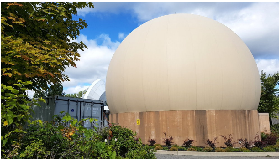
This radome at SSi Canada's offices in Kanata, Ont., encloses one of the satellite dishes the company uses to run its Qiniq and SSi Mobile networks. (File photo)
